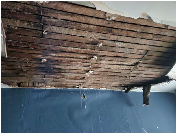
Large Conference Room – 2 nd Floor South Wall & Ceiling
