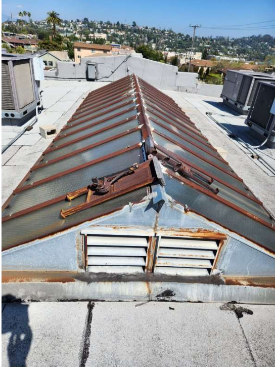
Upper South Roof Skylight (above stained glass ceiling of Sanctuary)
