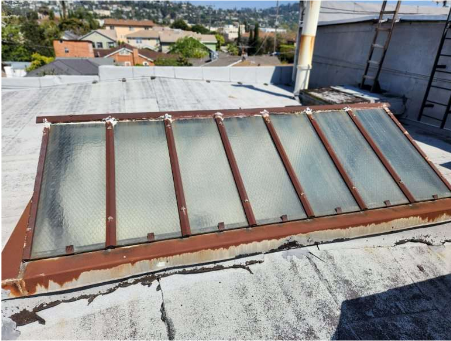
Lower North Roof Skylight (above stained-glass ceiling of Ryland Room)
