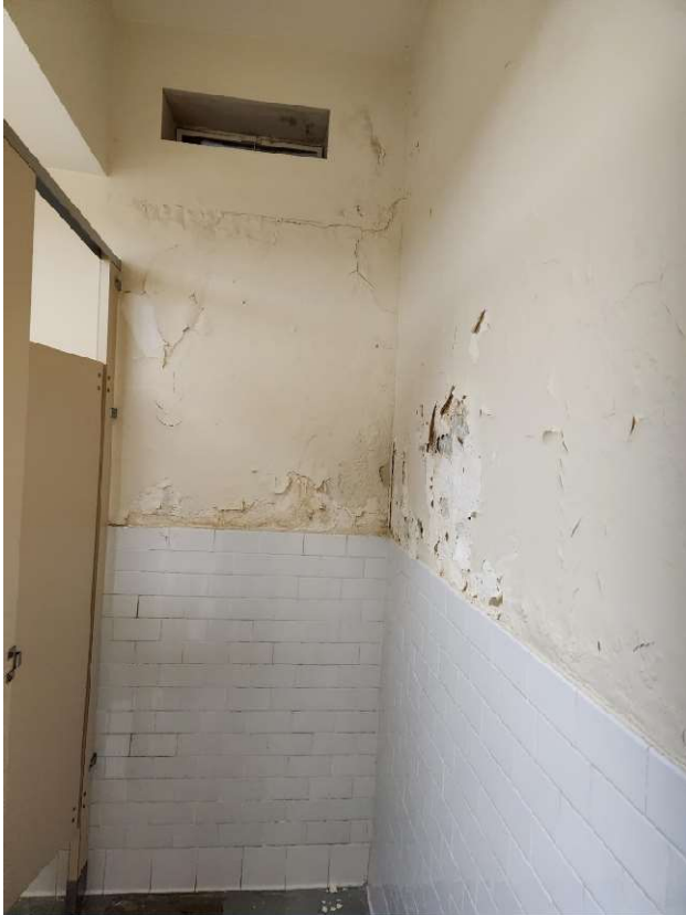
Basement Women's Restroom – Northwest Corner Walls
