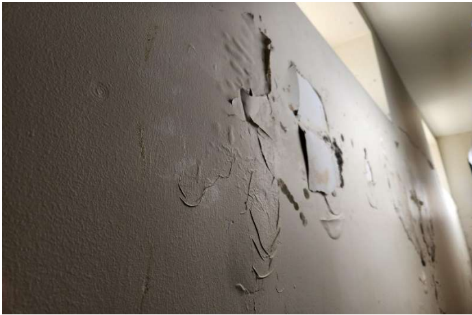
Fellowship Hall – East Wall
